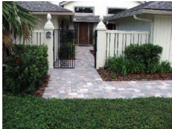
This walkway has been enhanced with the Oak Run-colored pavers in the Appian Stone shape and the "T" pattern.
